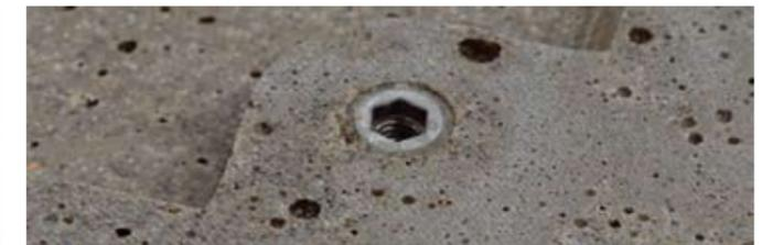
Our systems of hidden anchorage are on substructure in aluminium to norm DIN 18516 formed by vertical mountings, solidly berthed to the carrying structures of the building and horizontal mountings place as support of the slabs. The capacity of the metallic substructure holds account, for the determination of the vertical and horizontal cargo, of the weight of the slabs compared to variables as, height, shape, exposure of the building, actions of the wind and thermal cargo.
